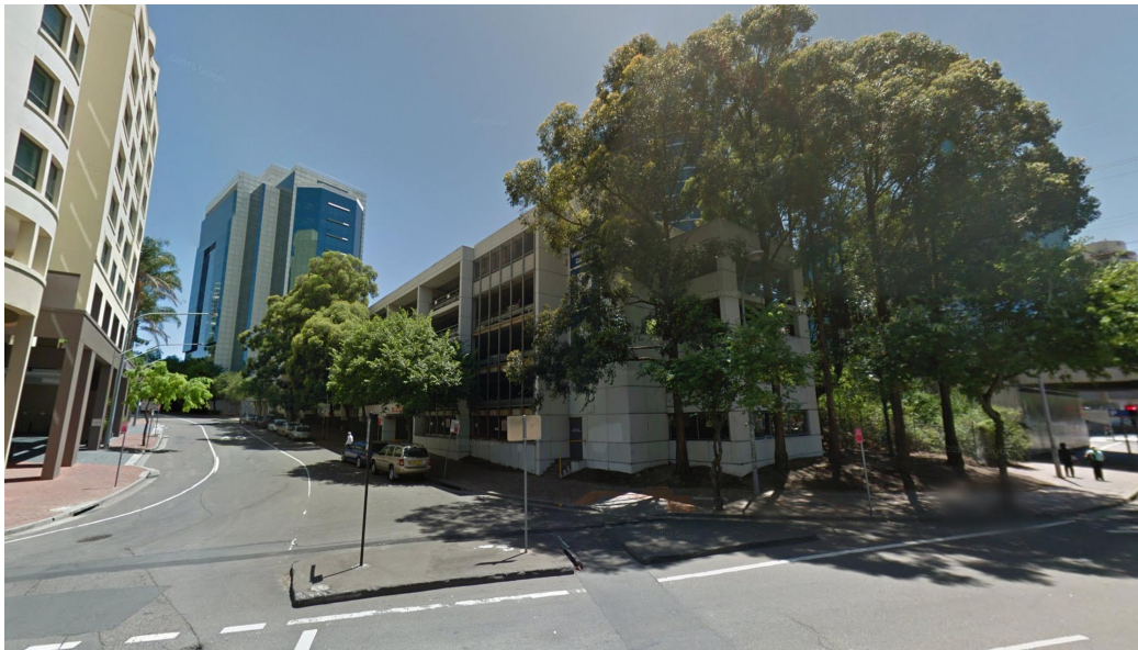
EXISTING CARPARK BUILDING
